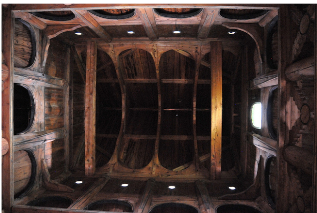
Figure 4. Borgund Stave Church roof interior, Borgund, Norway, 12th c. CE.
